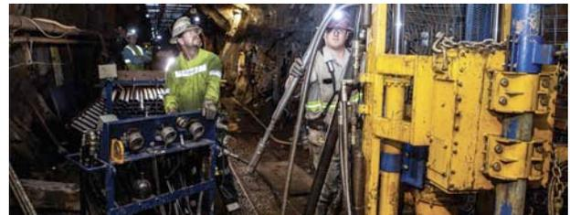
*Figure 7: Joel Carr (First Drilling) at left operates the controls of a drill rig in the west drift of the 4850 Level; Brad Burnett (right) reads the latch mechanism used to retrieve the core from the drill hole*
