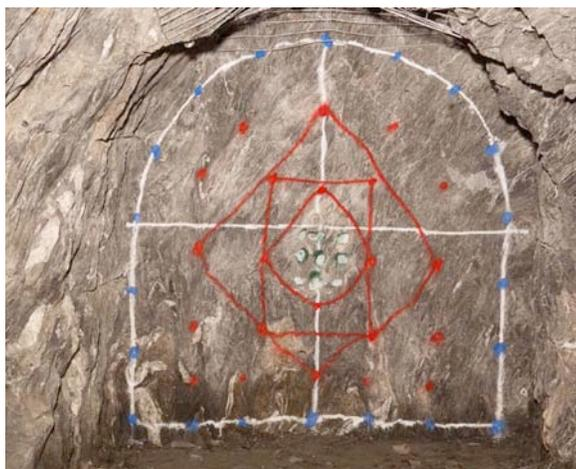
*Figure 5: This image illustrates the sequence in which a blast round happens*
