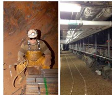
Figure 7: (Left) Bill Geffre prepares rock bolts for installation; (Right) Pipe installed in the West Drift runs from the Yates to the Ross Campus
