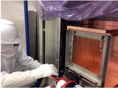
*Figure 3: Member of MAJORANA DEMONSTRATOR collaboration installs one of the inner copper shield boxes*
