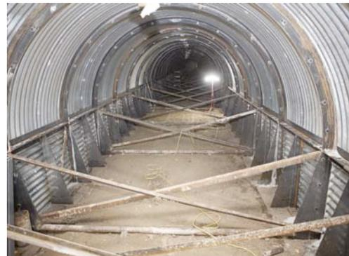
Figure 11: During the backfilling process, the tunnel was reinforced with supports
