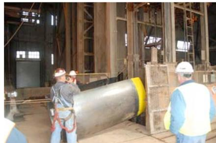
*Figure 4: Loading the mock load with slings attached to Yates south cage*
